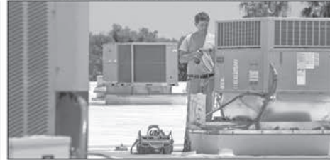
AIR CONDITIONING INSTALLS
