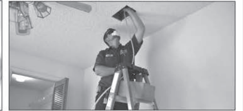
AIR CONDITIONING DUCT CLEANING
